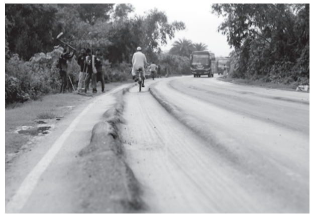
Figure 3. Rutting with high depth at Baromile (24°00'17.3"N 89°00'57.4"E)
