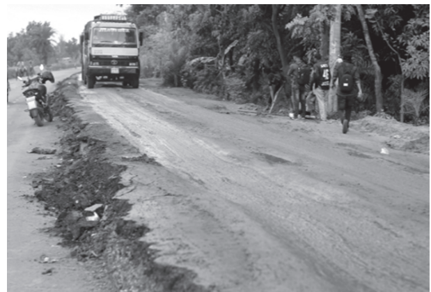
Figure 4. Rutting at Bahalbaria Bazar section (23°58'06.4"N 89°02'03.1"E)
