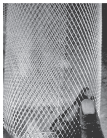
Figure 2. SSWM case preparation: tying with SSW (left), sewing with SSW (right)
